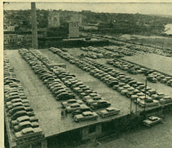
Parking for nearly 600 automobiles has been built right in the middle of the yards. The double-deck parking facilities are across the street in front of the Live Stock Exchange building.
