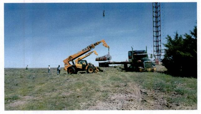
June 8, 2016 - All the rigging, preparations, and GIN pole are in place for an antenna lift.
